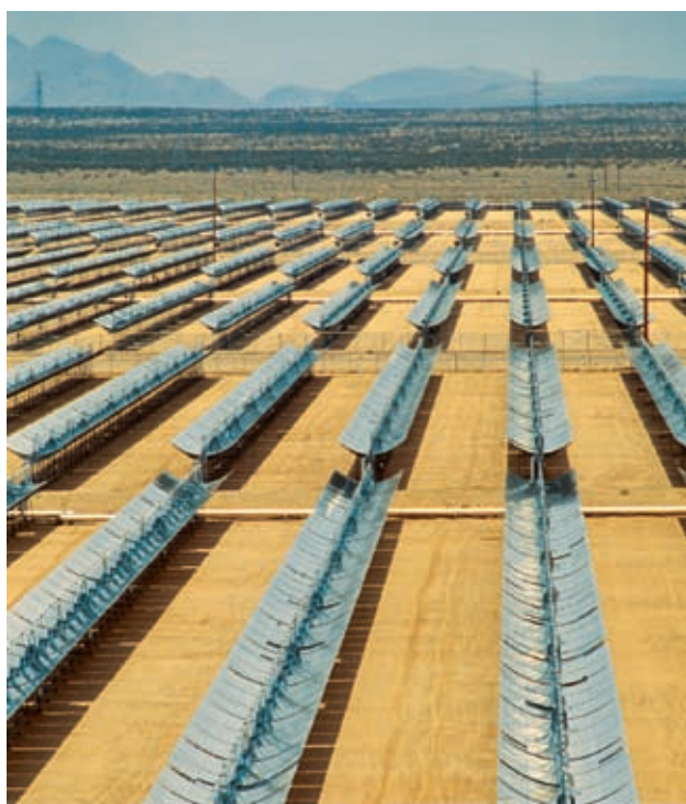
Solar Thermal Power Plant
